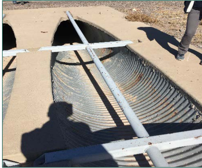
Photo 9: 2 X 48-inch CMP Culverts on the West Side of NM 26
