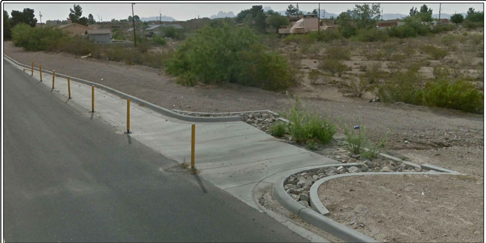
IMAGE 1: THE EXISTING RUNDOWN, ABOVE, IS LOCATED ON WESTMORE AVENUE. THE PROPOSED RUNDOWN, BELOW, HAS SIMILAR DESIGN FEATURES AND IS LOCATED ON WEBB ROAD. SEE BELOW FOR RUNDOWN LIMITS.
