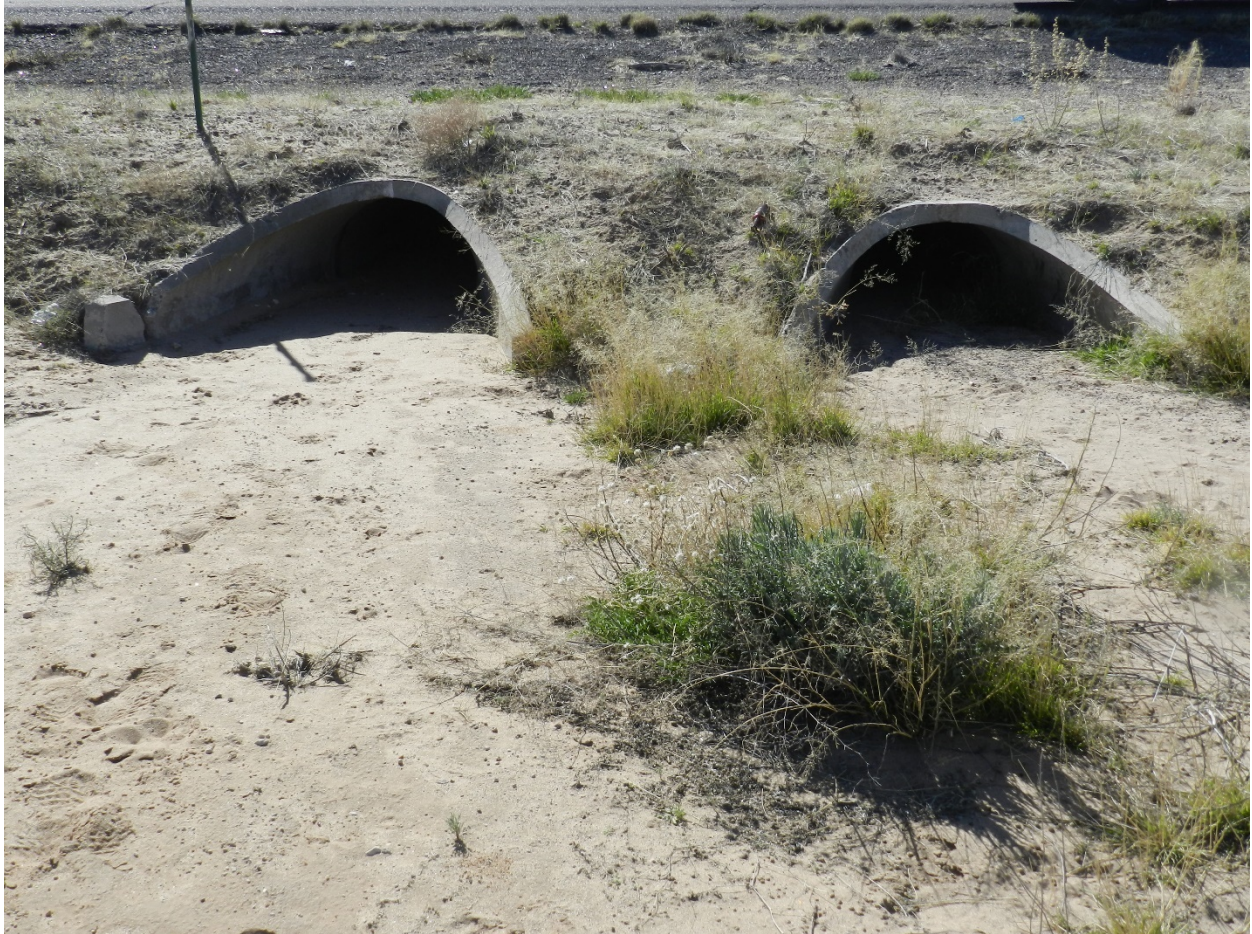
Photo 25: 2 – 24 inch RCP (NE9/NW4) inlet pipe located below I-25. Inlet has signs of sediment build up.
