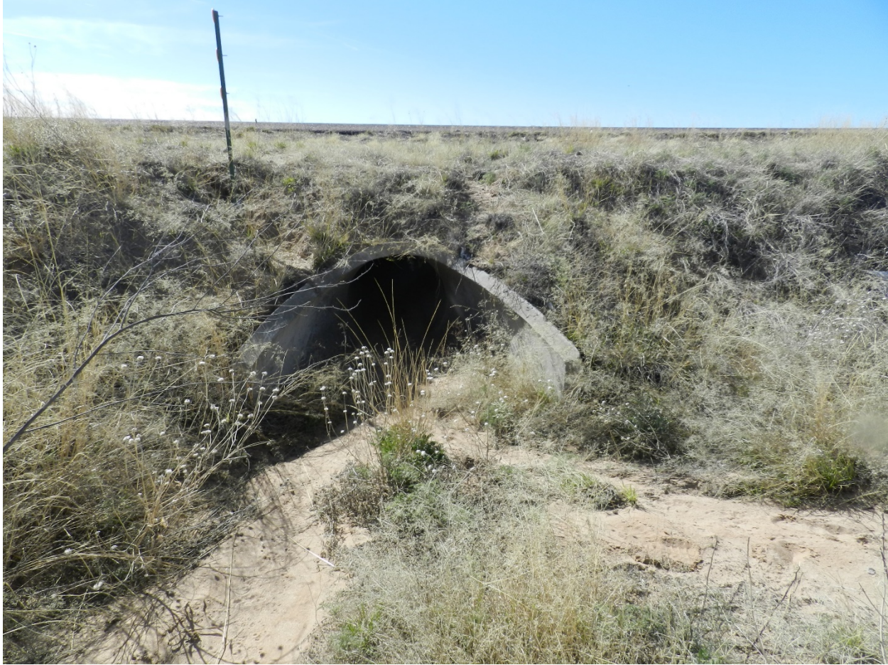
Photo 22: 1 – 30 inch RCP (NE6/NW7) inlet pipe located below I-25. Inlet has small signs of sediment build up.
