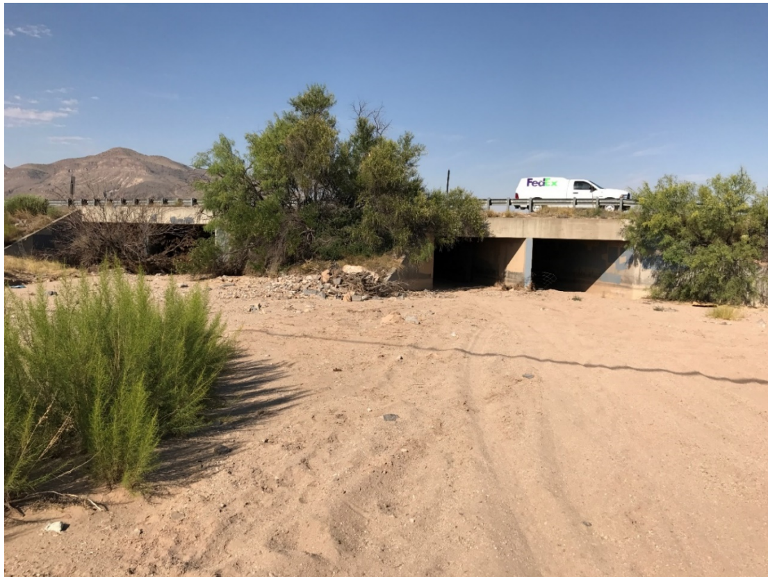
Photo 30: 4 – 10 ft. X 8 ft. CBC (SE3) located below I-25. Inlet has some signs of sediment build up.
