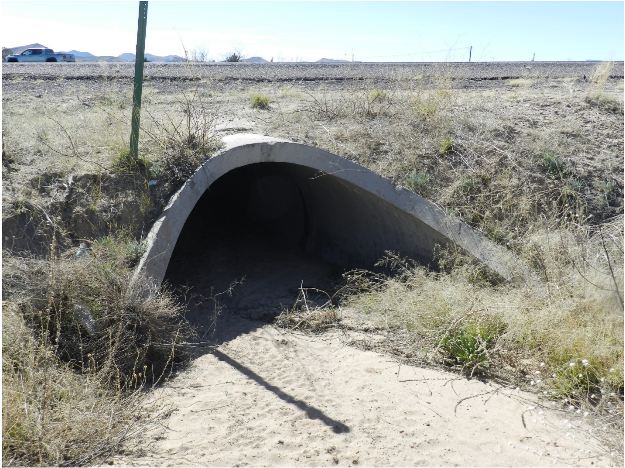
Photo 19: 1 – 54 inch RCP (NE2) inlet pipe located below I-25. Inlet has signs of sediment build up.
