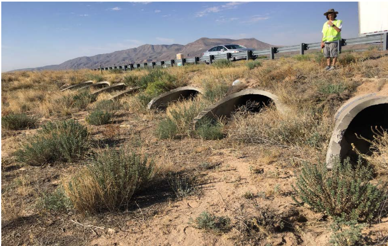
Photo 2: 8 - 36 inch RCP pipe located also on the east side of I-25. Partially filled with sediment from upstream. (NE 5.2/NW8)
