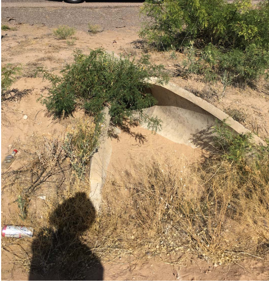
Photo 3: 1 – 30 inch RCP pipe located on the East side of I-25. Inlet was clean with very little sediment. (NE8)
