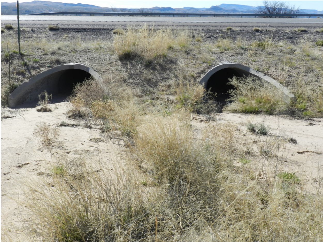
Photo 26: 2 – 24 inch RCP (NE10) inlet pipe located below I-25. Inlet has signs of sediment build up.
