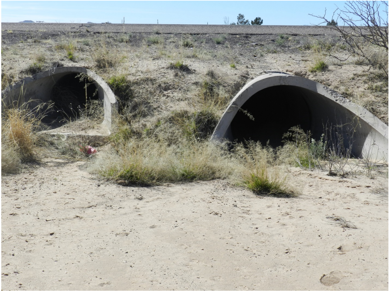
Photo 18: 1 – 54 inch RCP (NE1.1) and 1 – 30 inch RCP (NE1.2) inlet pipes. Inlets have small signs of sediment build up and go under I-25.
