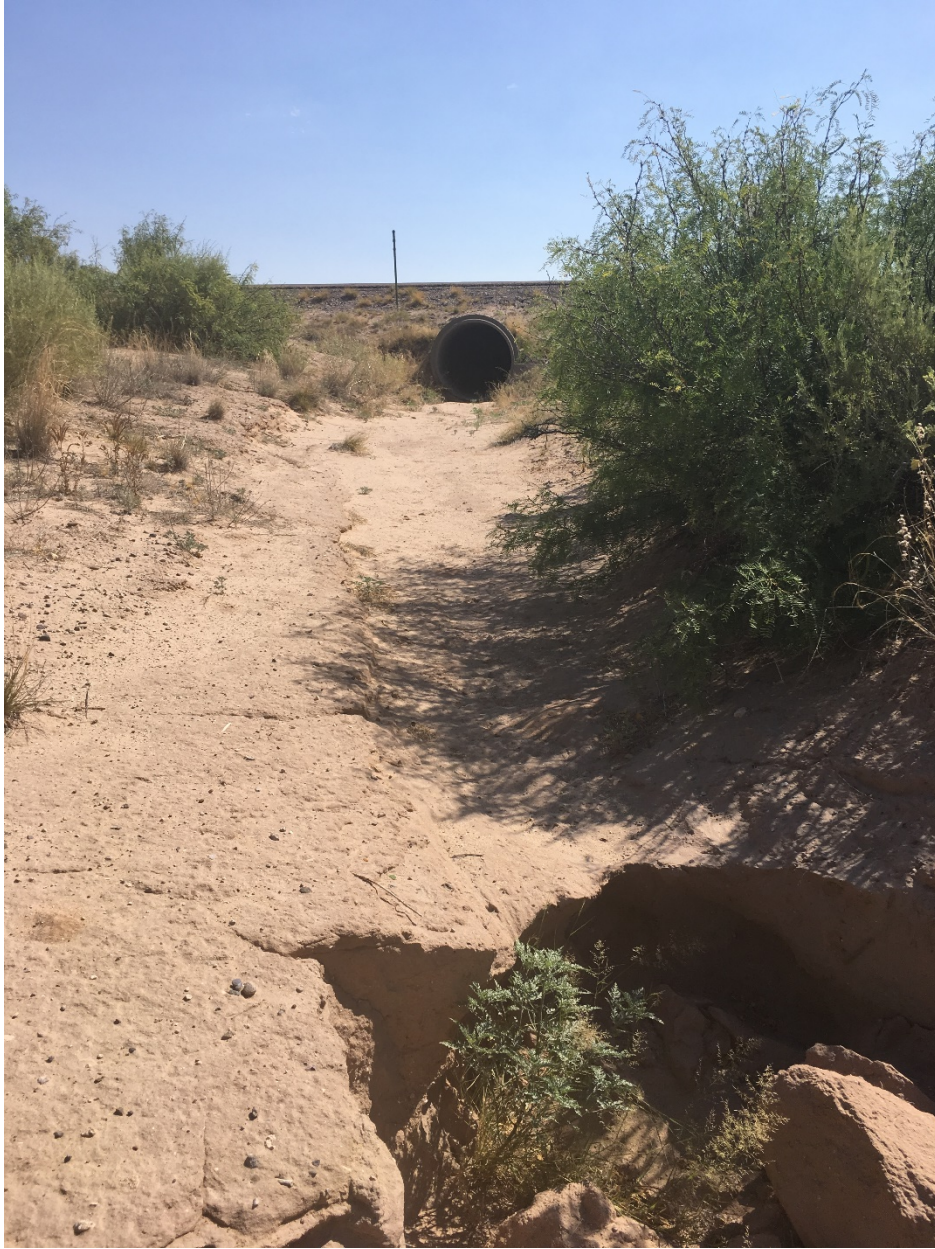
Photo 9: 1 – 54 inch RCP pipe located on the West side of I-25. Inlet was clean and no sign of being filled with sediment. (NW11)
