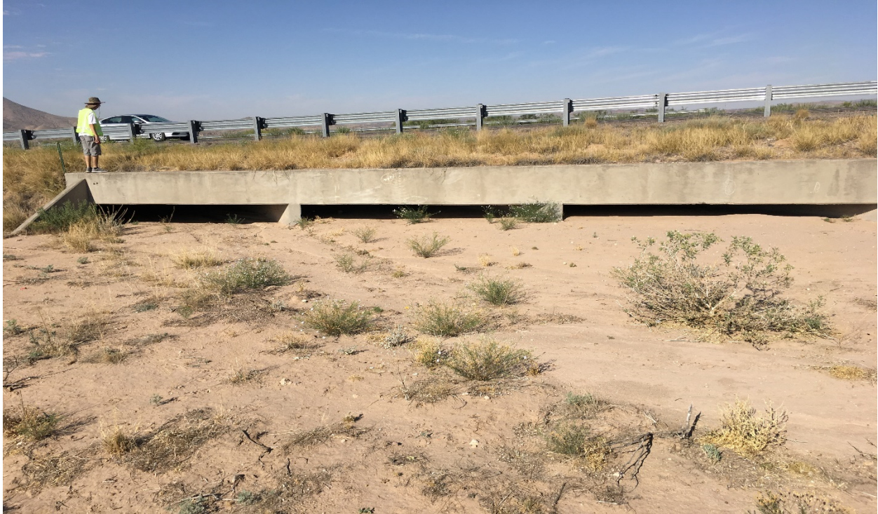
Photo 1: 4 - 1.5' x 14' CBC pipe located on the east side of I-25. Flow is restricted due to the box culvert being filled with sediment. (NE 5.1/NW8)
