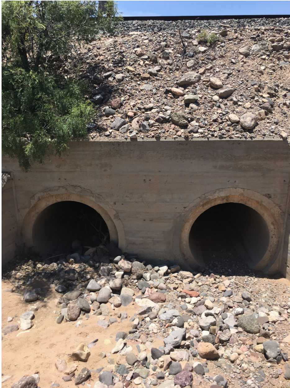
Photo 14: 2 – 36 inch RCP pipe located under the Railroad going East to West. Inlets have small amounts of sediment present in pipes. (Railroad 1)
