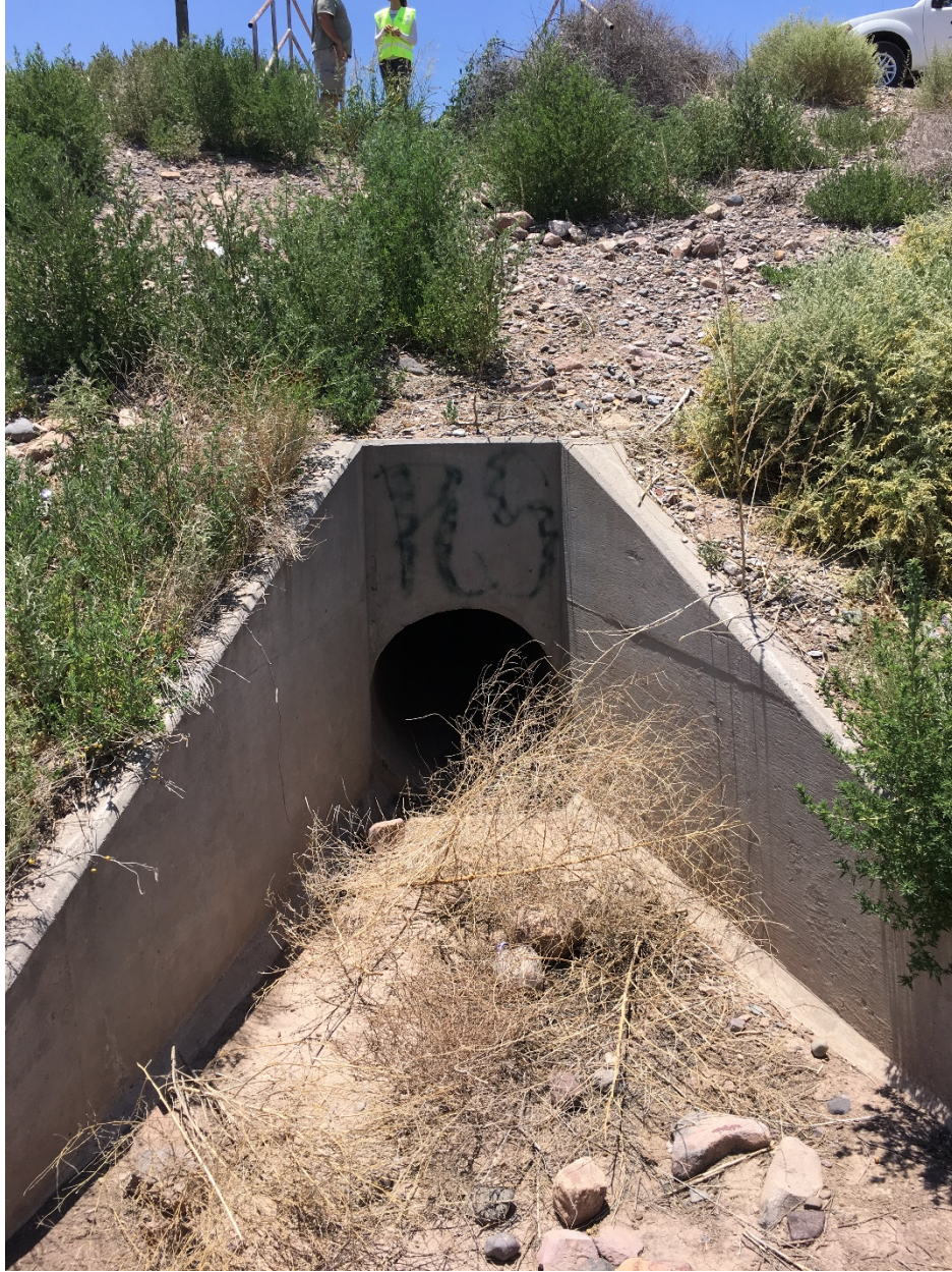
Photo 17: Lucero Dam principle spillway invert within pond bottom.
