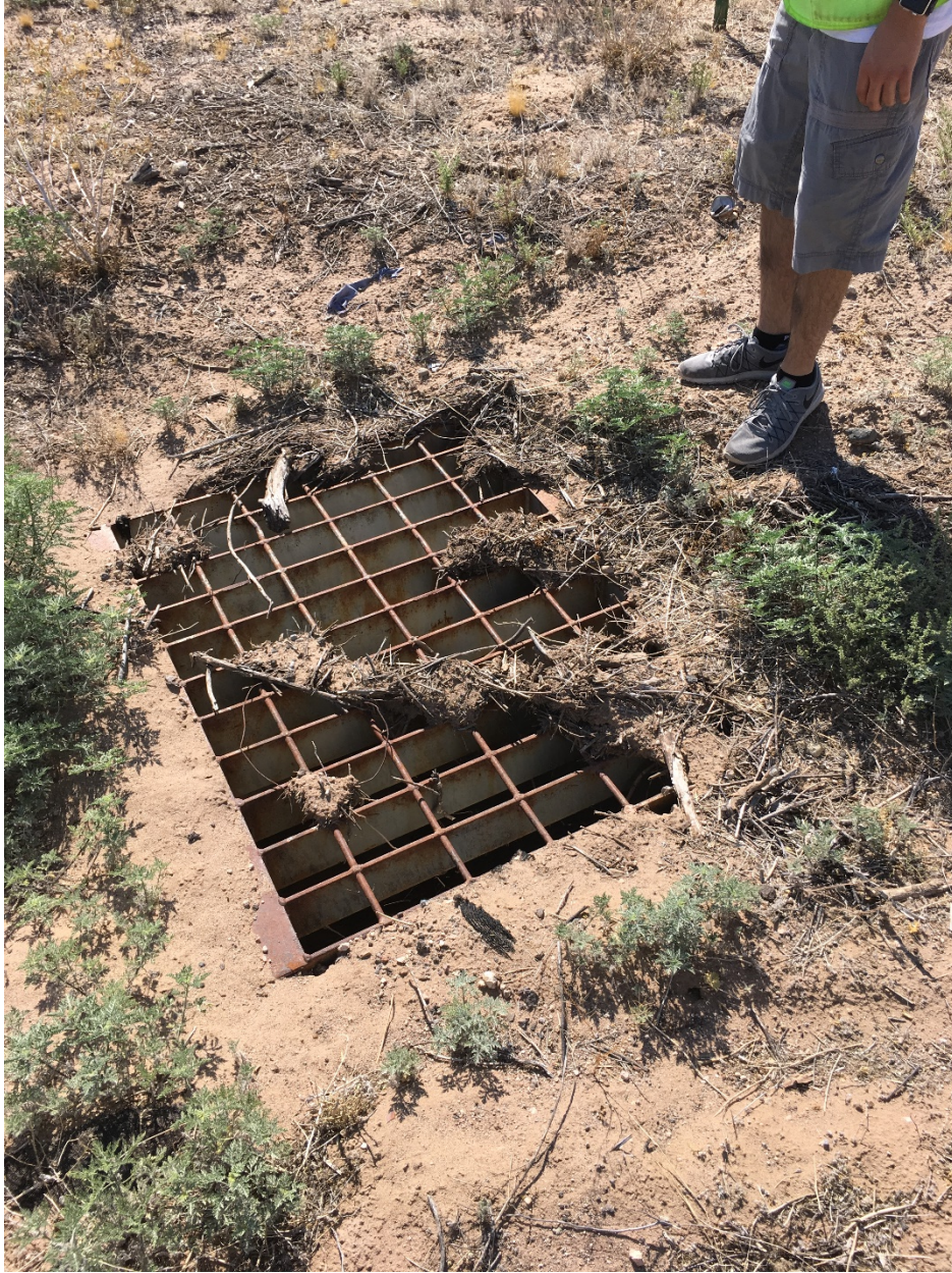
Photo 6: Median drop inlet into culvert NE 11 located in the median of I-25.
