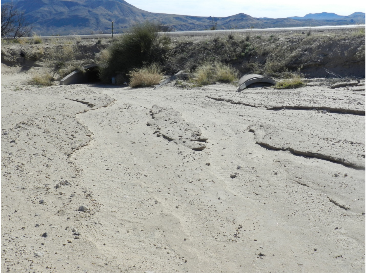
Photo 27: 3 – 36 inch RCP (NE11/NW3) inlet pipe located below I-25. Two of the three inlets are filled with sediment, and the third has sediment build up.
