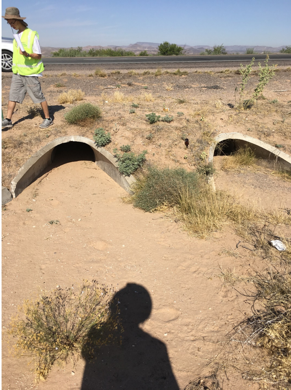
Photo 5: 2 – 24 inch RCP pipe located on the East side of I-25. Inlet was partially filled with sediment. (NE9)
