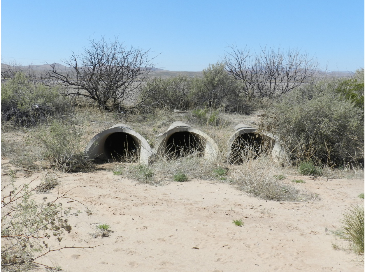
Photo 31: 3 – 30 inch RCP (SE2/SW1) inlet pipe located below I-25. Inlet has some signs of sediment build up.
