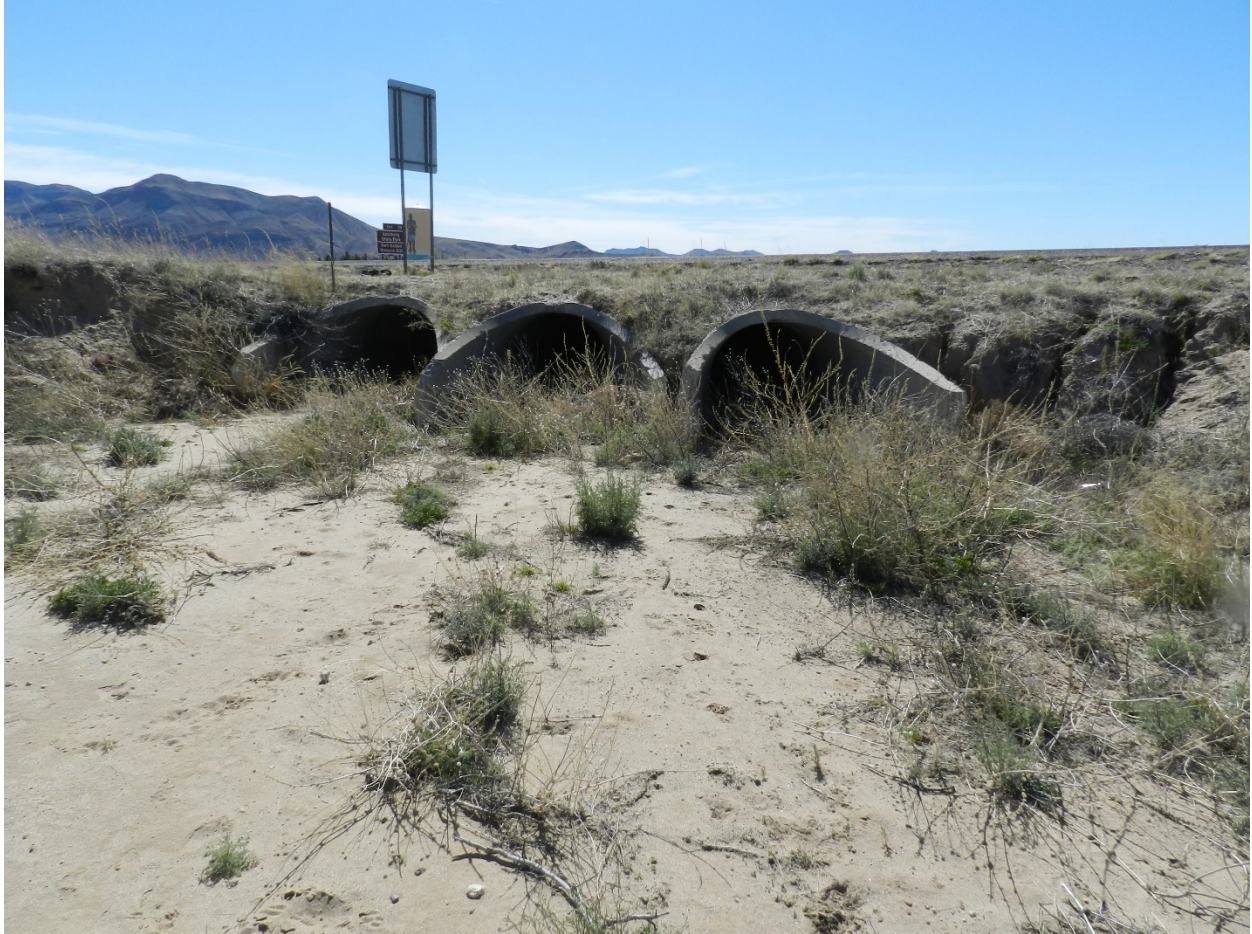
Photo 21: 3 – 48 inch RCP (NE4/NW9) inlet pipe located below I-25. Inlet has small signs of sediment build up.
