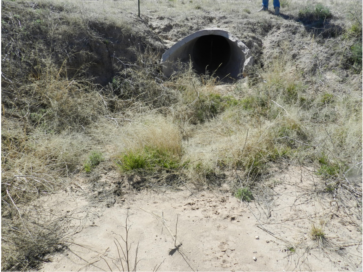
Photo 20: 1 – 30 inch RCP (NE3/NW10) inlet pipe located below I-25. Inlet has small signs of sediment build up.
