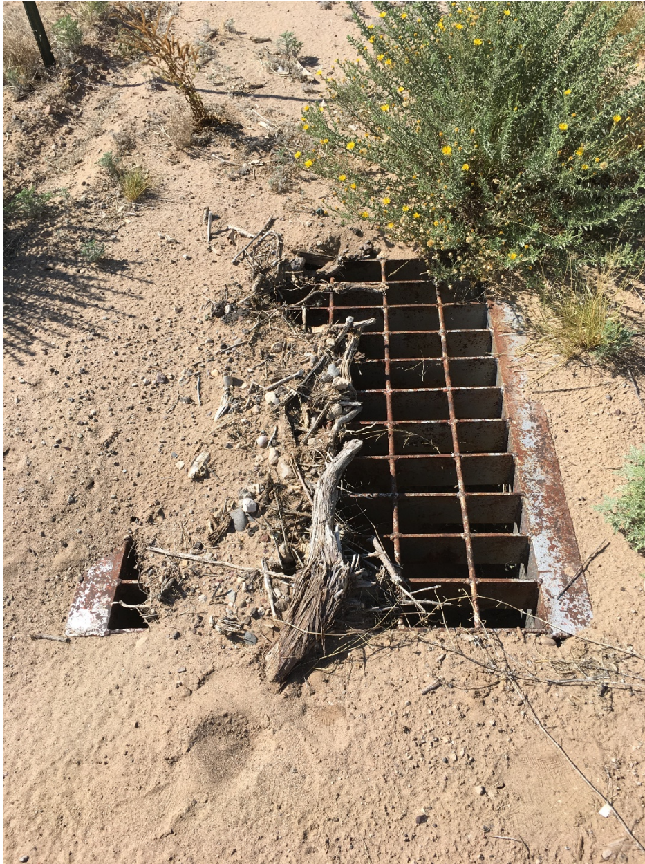
Photo 7: Median drop inlet into culvert NE 3 located in the median of I-25. Drop inlet partially blocked by sediment and debris.
