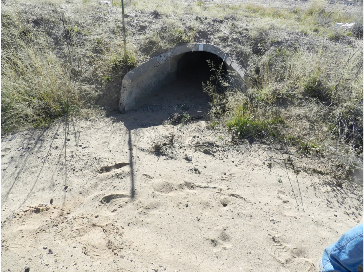
Photo 28: 1 – 30 inch RCP (NE12/NW2) inlet pipe located below I-25. Inlet has signs of sediment build up.
