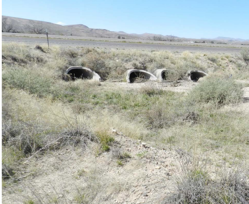
Photo 29: 4 – 36 inch RCP (SE4) inlet pipe located below I-25. Inlet has signs of sediment build up.
