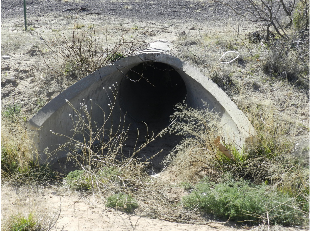
Photo 24: 1 – 30 inch RCP (NE8/NW5) inlet pipe located below I-25. Inlet has a crack at the top of the pipe.
