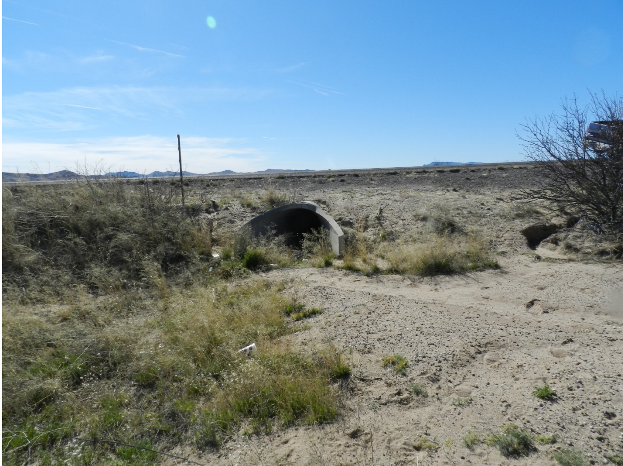
Photo 23: 1 – 30 inch RCP (NE7/NW6) inlet pipe located below I-25. Inlet has small signs of sediment build up.
