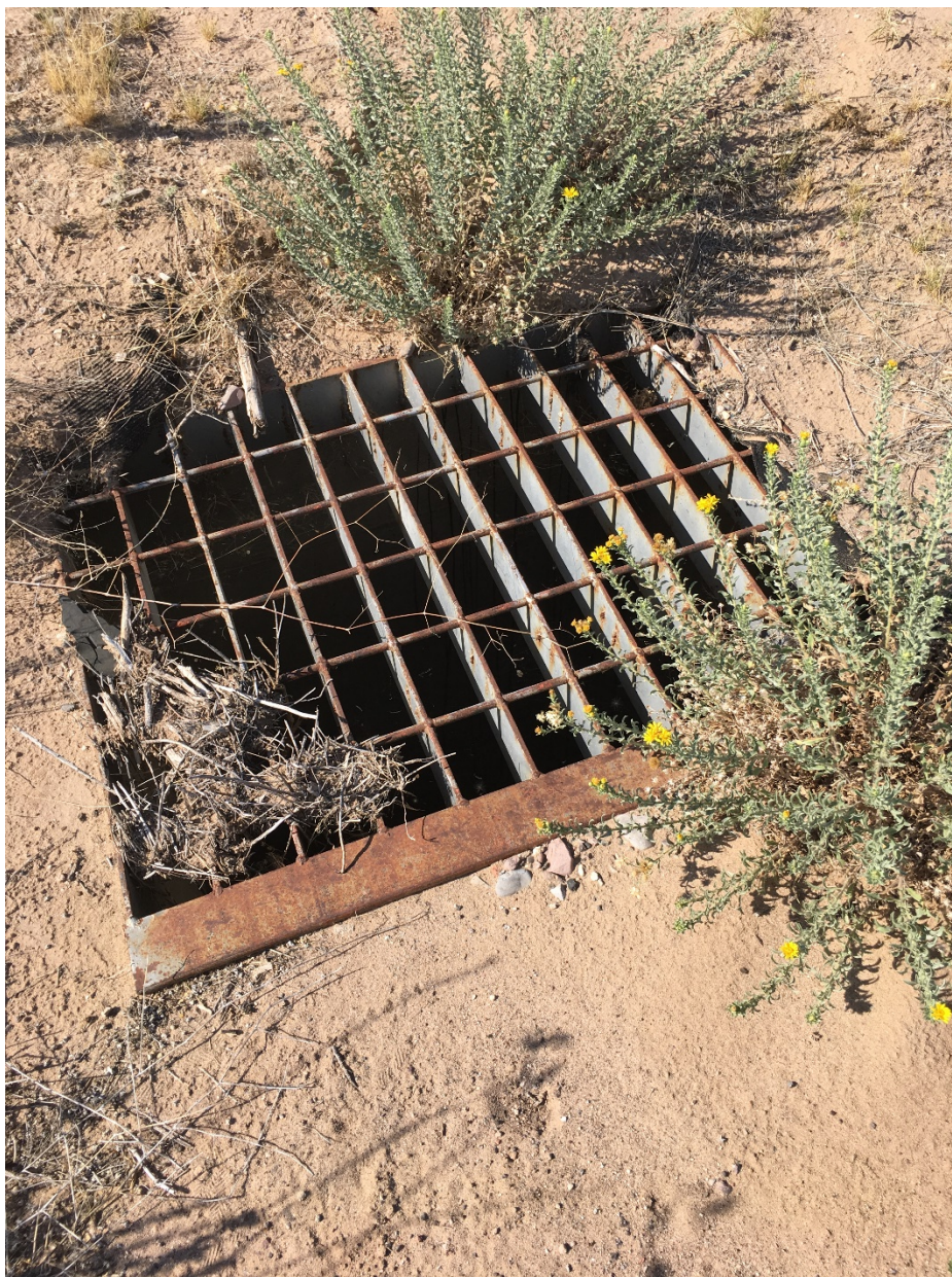
Photo 4: Median drop inlet into culvert NE 8 located in the median of I-25.
