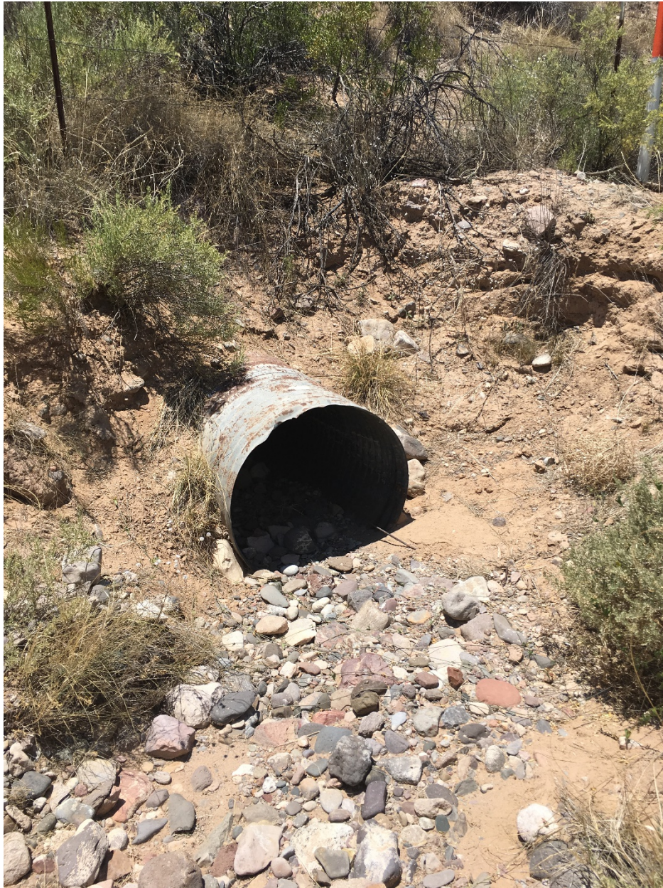
Photo 15: 1 – 30 inch CMP inlet pipe located below State Park Road Inlet has small signs of sediment build up. (Railroad 2)
