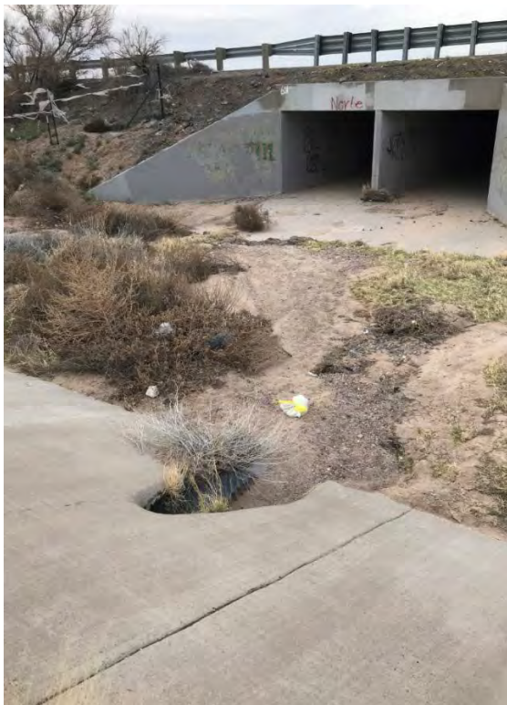
Figure 8: Culvert 1 (1 @ 24" CMP) under east frontage road (near CBCs) Downstream: is shown here (full of debris). Upstream is shown above.
