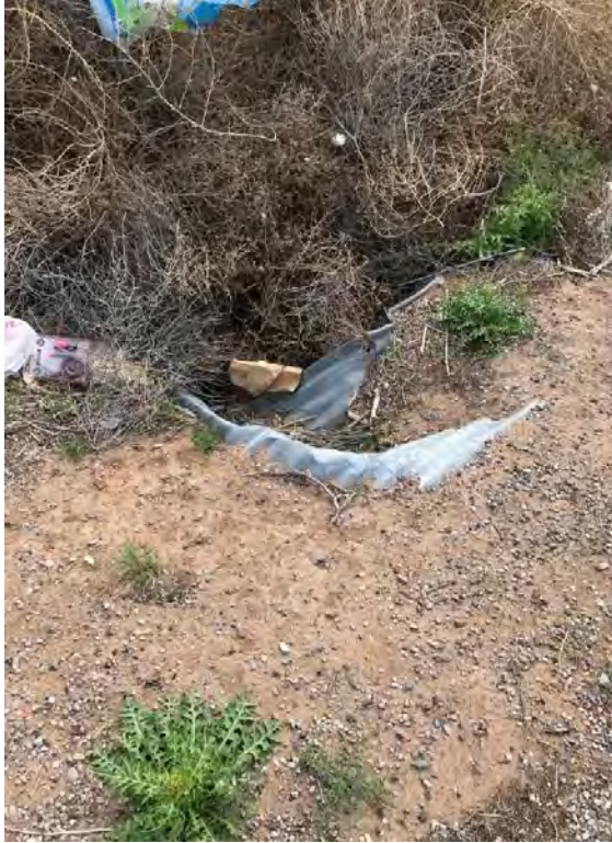
Figure 5: Culvert under west frontage road downstream of Culvert C5. It is supposed to be 36" CMP but upstream is deflected so the culvert rise is reduced to approximately 24"
