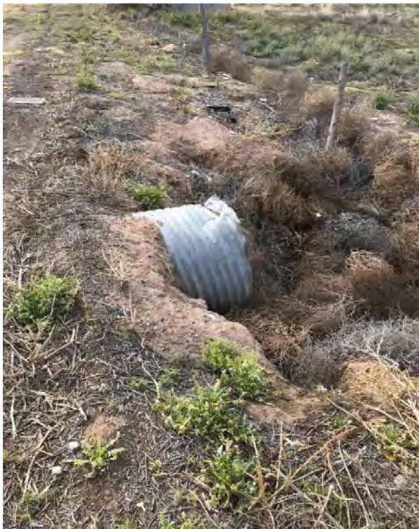
Figure 4: Culvert under west frontage road downstream of Culvert C5. It is supposed to be 36" CMP but upstream is deflected so the culvert rise is reduced to approximately 24" (see next picture).
