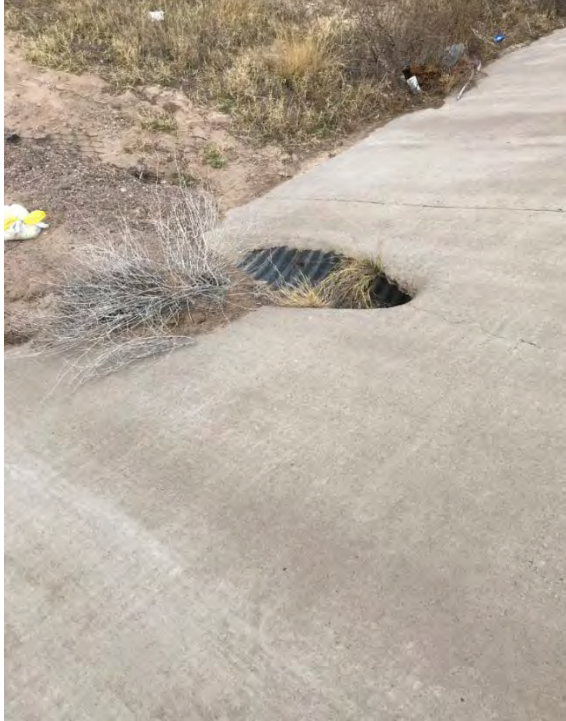
Figure 7: Culvert 1 ( 1 @ 24" CMP) under east frontage road (near CBCs). Upstream: full of debris, hard to find! Downstream: is shown above
