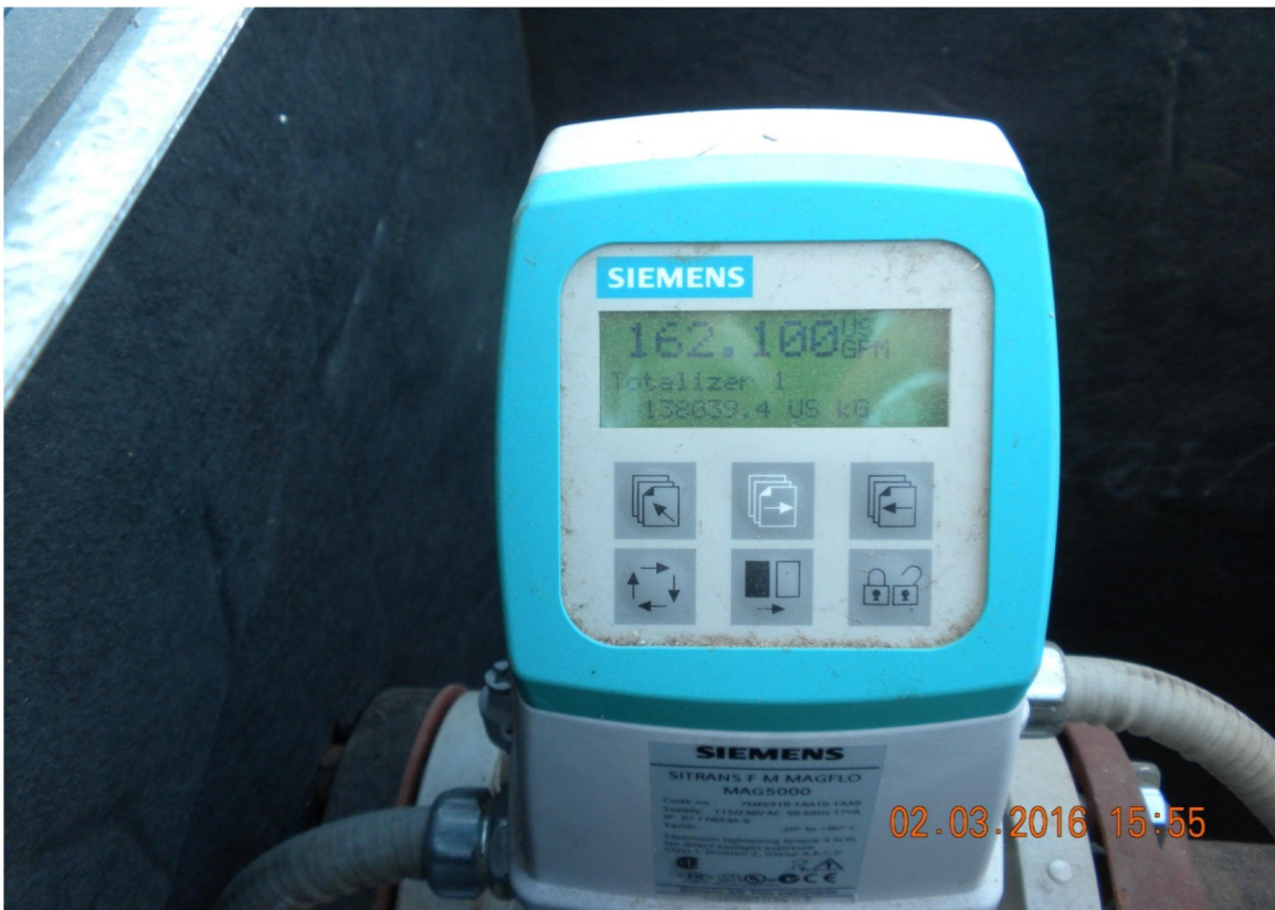
Close-up view of the water discharge flow meter at CLC Well 27 indicating an extraction rate of approximately 162 gallons per minute (West view).
